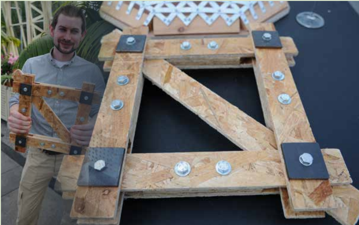
Innovative use of OSB by Matt Collins, University of Limerick, the winner of the Engineering Award at the Wood Marketing Federation Student Awards. He explored a grid shell concept to produce large load bearing spans using oriented strand board
