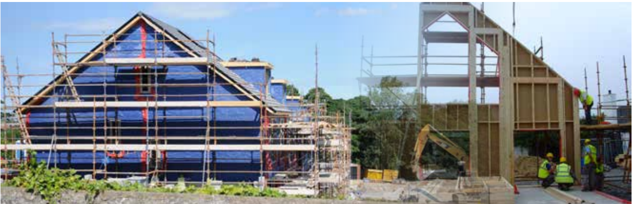
New timber frame houses being constructed in Ireland
