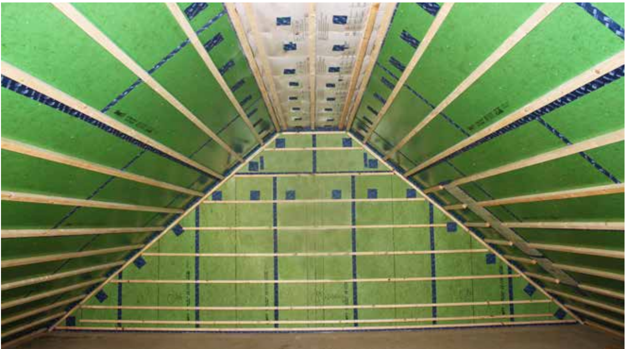
SMARTPLY PROPASSIV used on the construction of a passive house.
